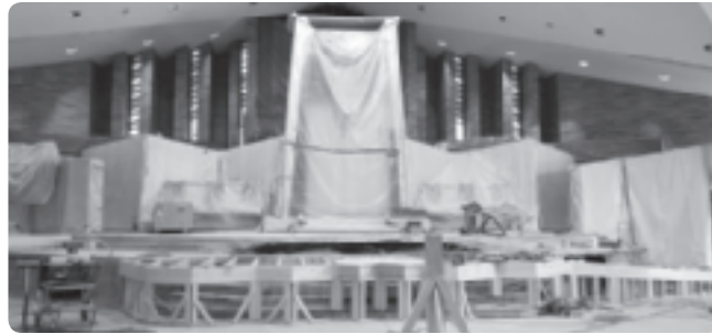
New bimah and ramps are being framed.
